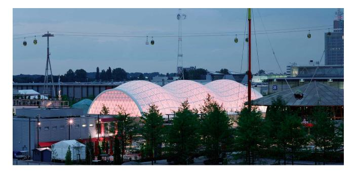
The theme for the 2000 Hannover Expo was sustainability, so a completely recyclable pavilion was designed. The pavilion took the form of a three-dimensionally curved, grid-shell tunnel arch composed of paper tubes connected together by fabric tape and reinforced by wooden ladder arches. This frame was covered by a membrane of fire resistant paper.
