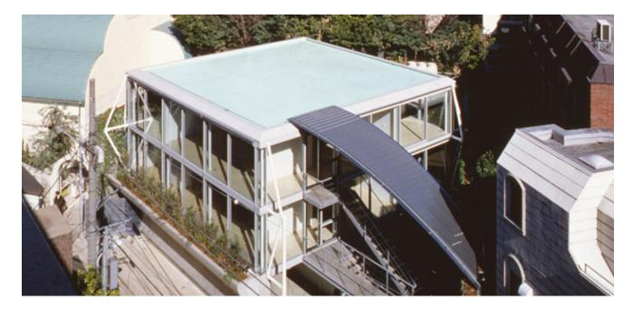
The three-storied glass cube is connected at three corners to a full height ivy screen, which functions as the primary structural support, thus the main characteristic of the ivy plant which is dependant on a separate structure becomes the main characteristic of the building, depending on the ivy screen. Because the ivy screen carries the lateral loads of the main building, the size of the interior columns was minimized to increase spatial flexibility.
