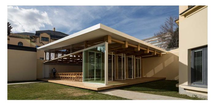
The pavilion is composed of a L-shape existing concrete wall, 6 paper tubes columns and a paper tubes truss roof sitting on top. The paper tubes are made of recycled paper and manufactured locally in Pina de Ebro (Zaragoza, Spain). For educational purposes, architectural students participated in assembling the Paper tube trusses together with the contractor.
